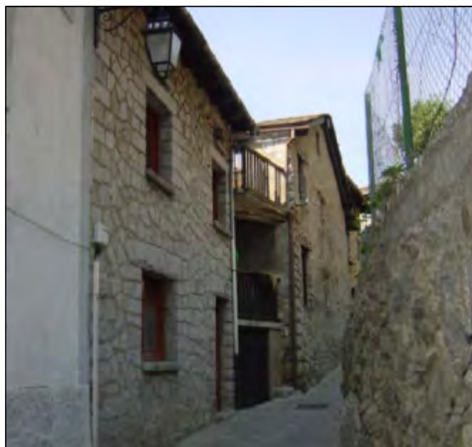
CARRER MAJOR, Nº17
