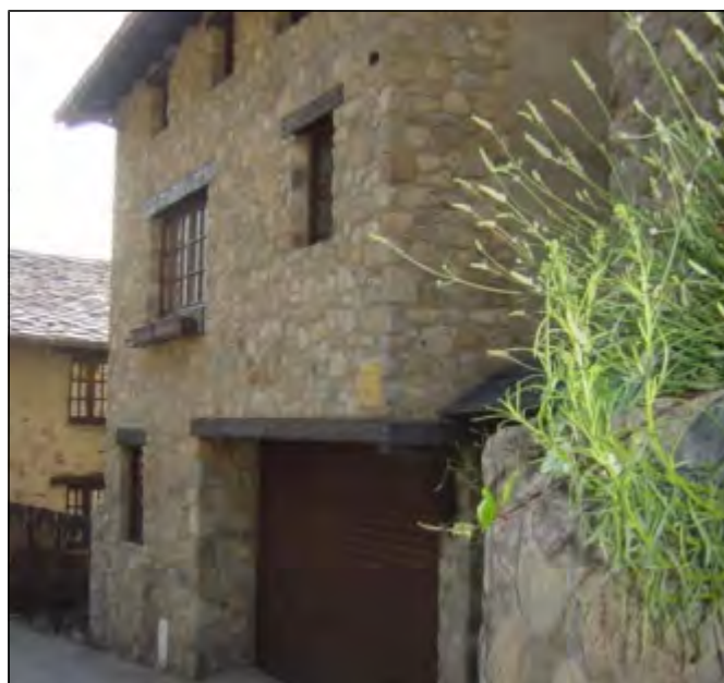
CARRER MAJOR, Nº21
